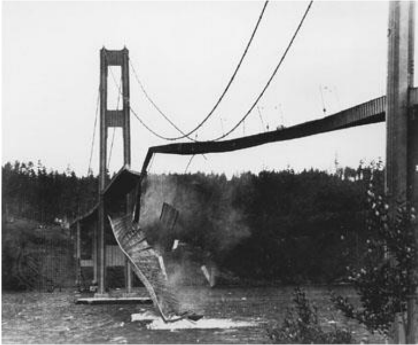
Collapse of Tacoma Narrows Bridge (1940)
